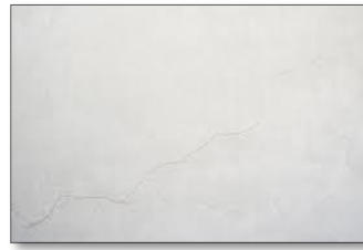
Hairline Cracks
